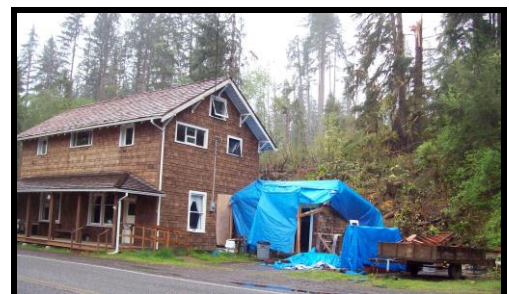
Today...Work in progress.
