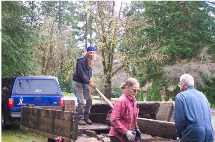
Brian, Brooke and John unloading railroad ties
